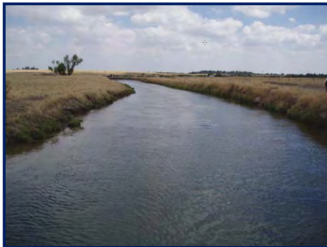
Figure 3-3. North Main Canal.
