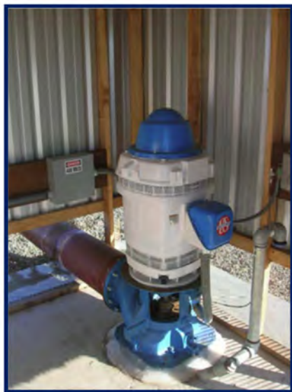
Figure 4-5. OID Irrigation Well.
