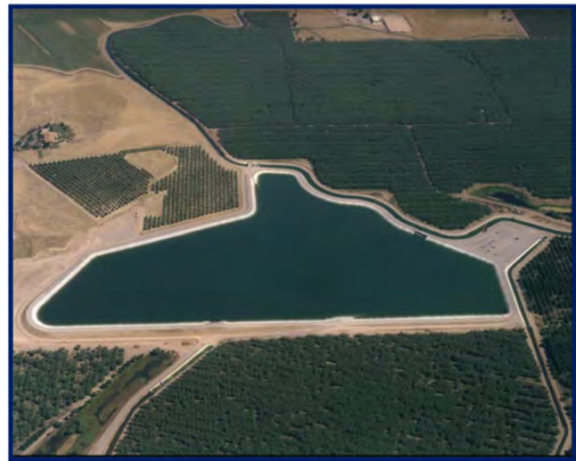
Figure 3-4. North Side Regulating Reservoir.
