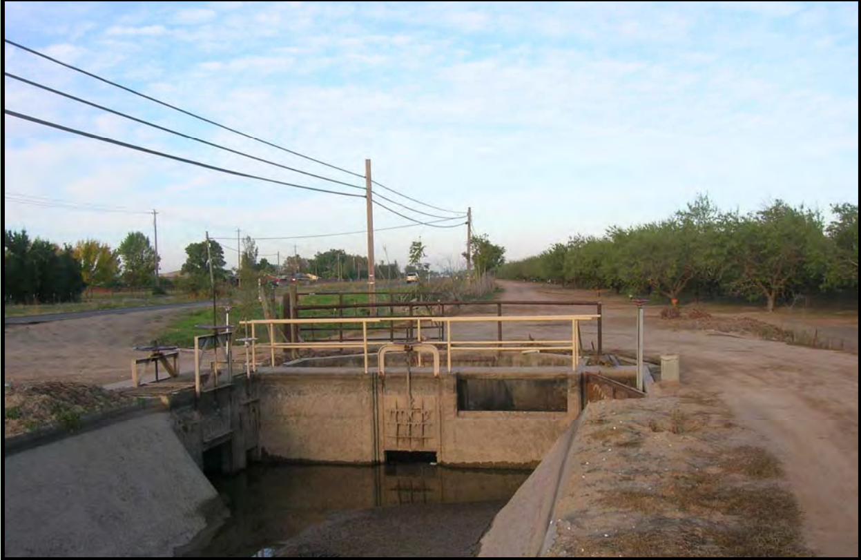
Burnett-River Road Diversion Structure Automation Project
