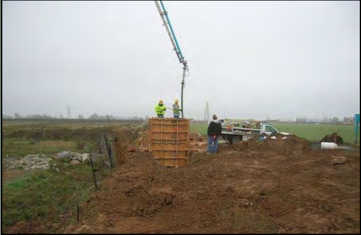
Southwest Pipeline Replacement Project
