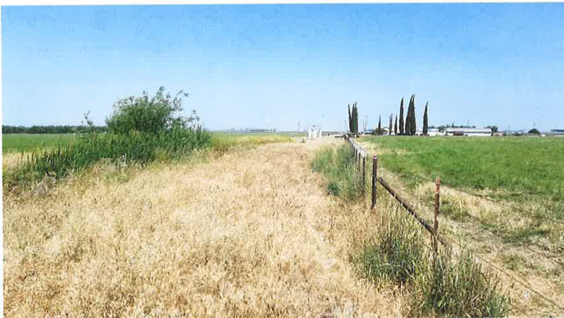
Looking east towards control structure within APN: 014-005-008 with historical point of delivery along the south bank of the Brichetto Lateral near the shared property line of APNs: 014-005-003 and 014-005-008.
