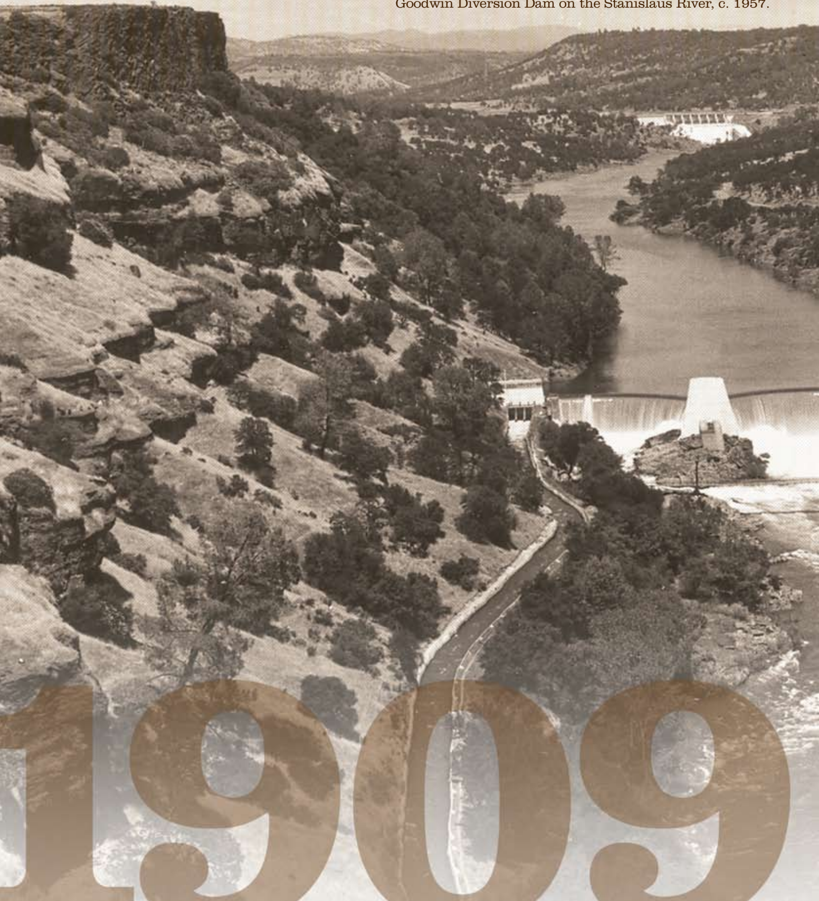
Goodwin Diversion Dam on the Stanislaus River, c. 1957.
