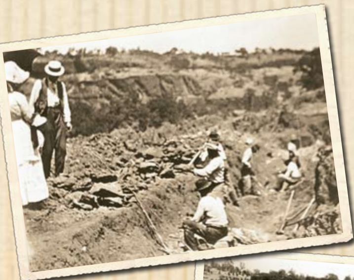
▲ Digging and enlarging the irrigation canals for the construction of the Oakdale Irrigation District in 1910.
