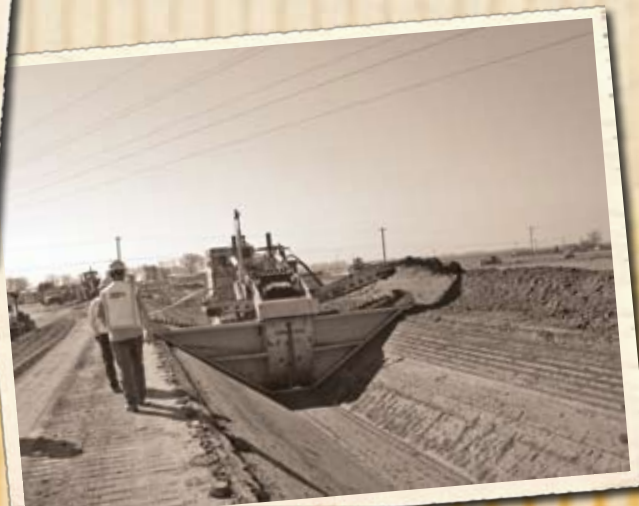
Rehabilitation of the OID distribution system is underway.
