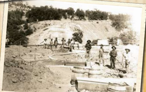
◀ Construction work on the canal near Knight's Ferry. 1910.
