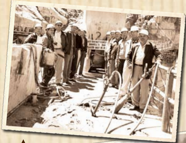
▲ The last bucket on Donnells Dam, May 15, 1957.
