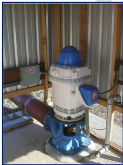
Figure 4-5. OID Irrigation Well.
