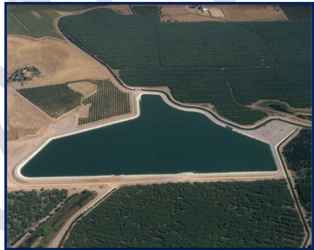
Figure 3-4. North Side Regulating Reservoir.
