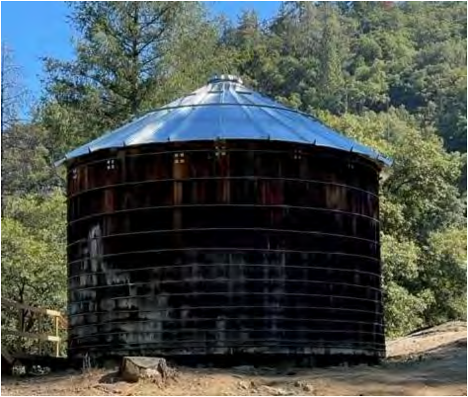
Beardsley Water Tank Roof
