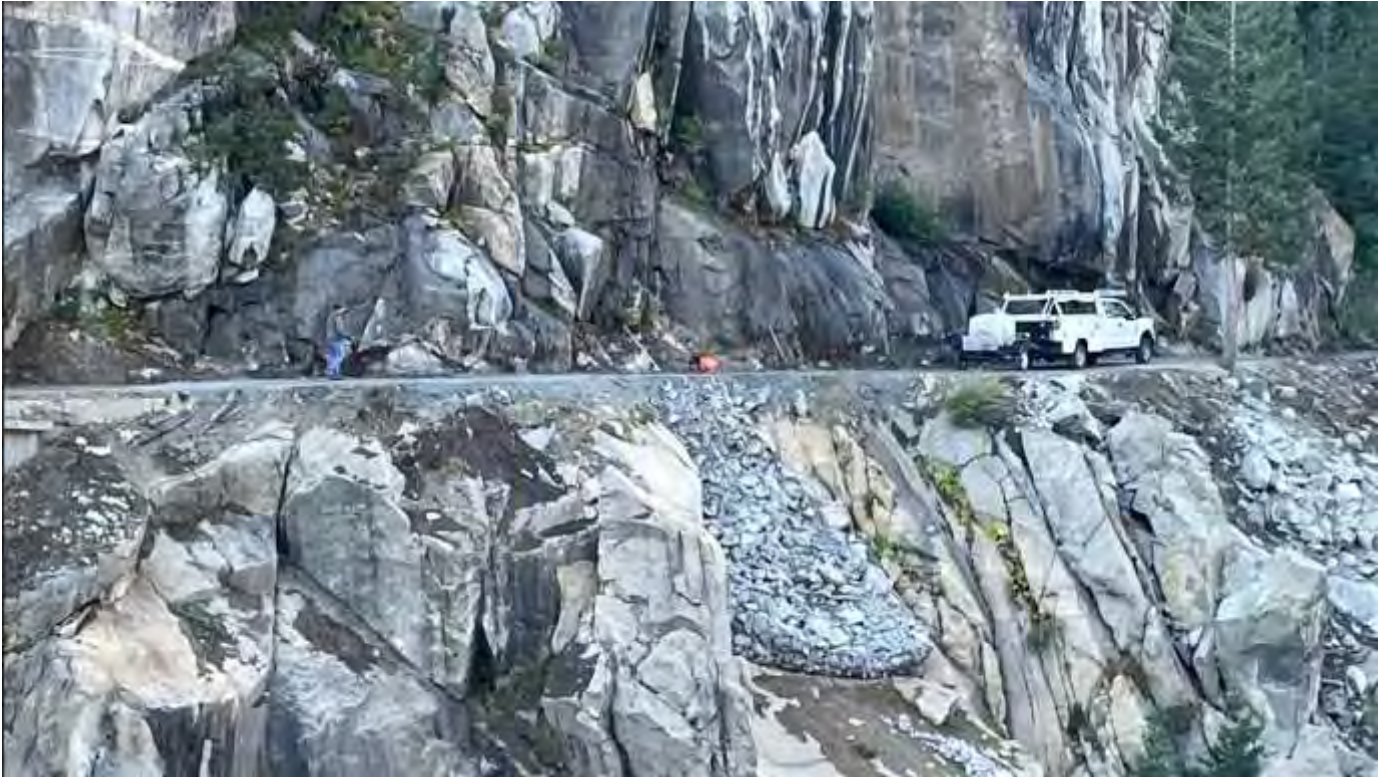
FEMA Site 5- Sink Hole Repair
