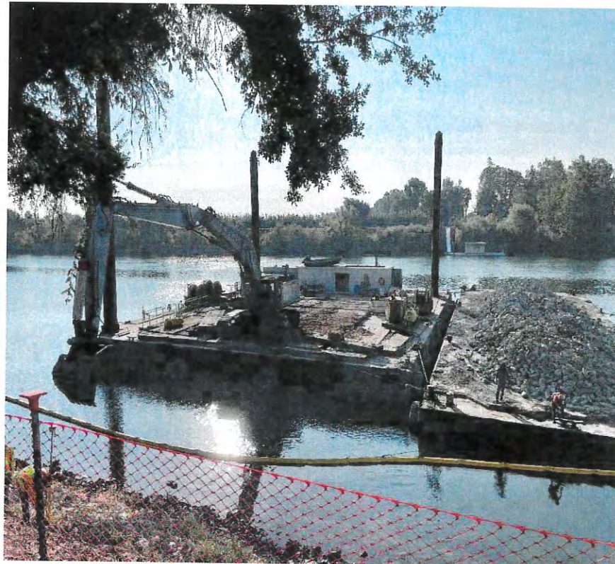
Figure 9 depicts an excavator placing riprap on a recent SMCI project.
