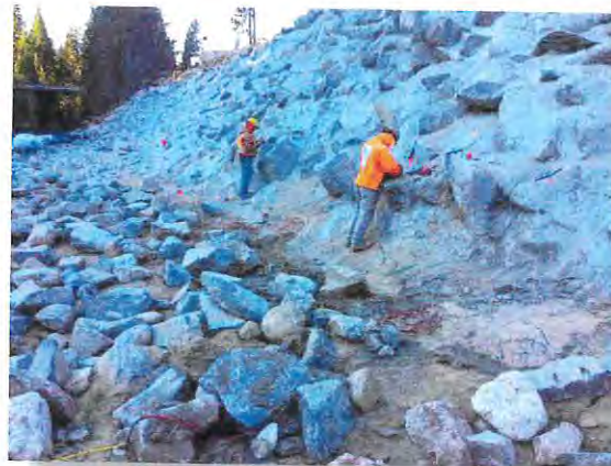
RSP - Eastwood Visitors Center Bank Stabilization
