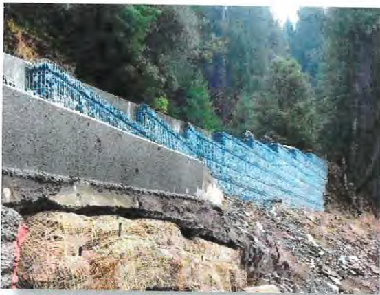
MSE Wall – Brush Creek Boat Ramp
