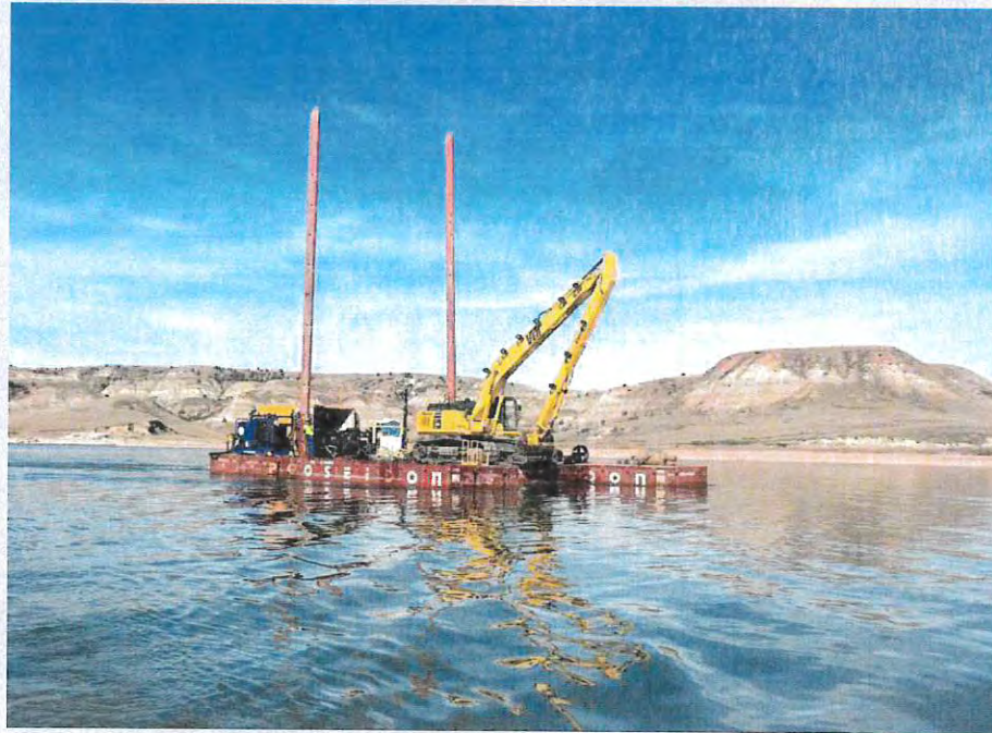
Figure 1 depicts a fully assembled flexifloat pontoon system.
