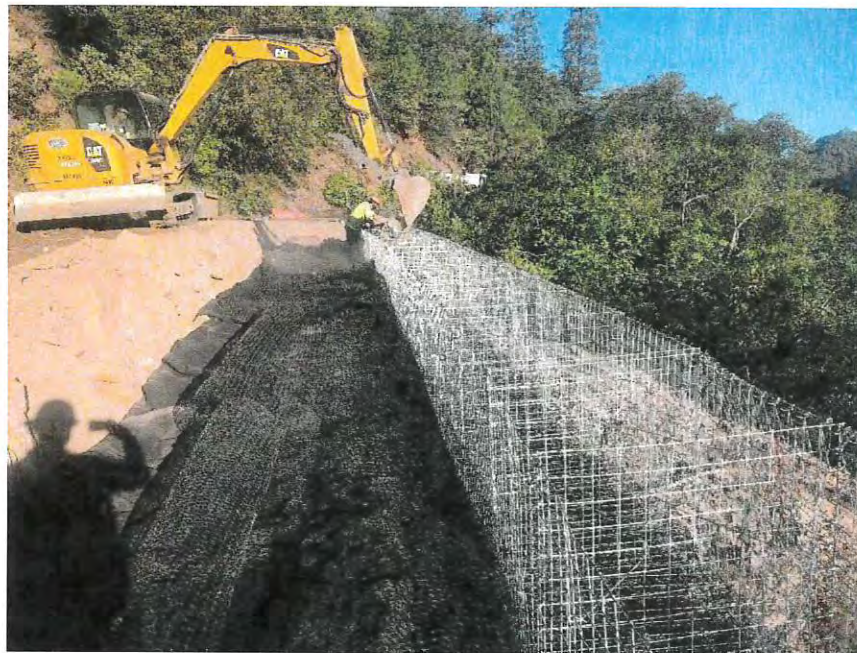
Figure 10 depicts a gabion basket installation on a recent SMCI project.
