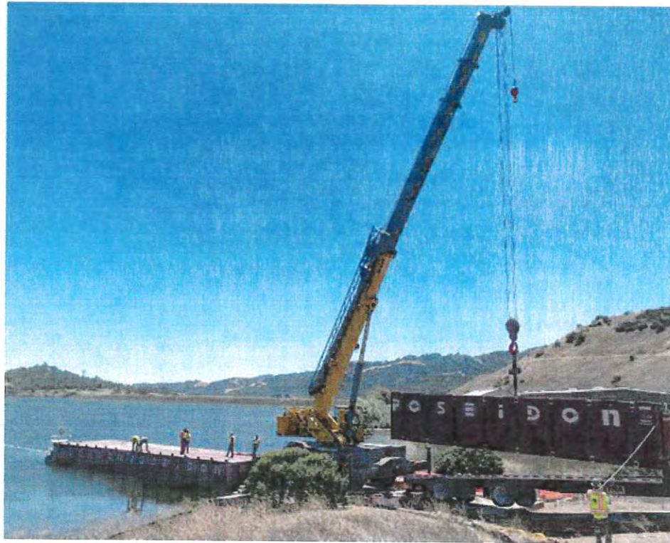
Figure 3 depicts the assembly of pontoons on a recent SMCI project.
