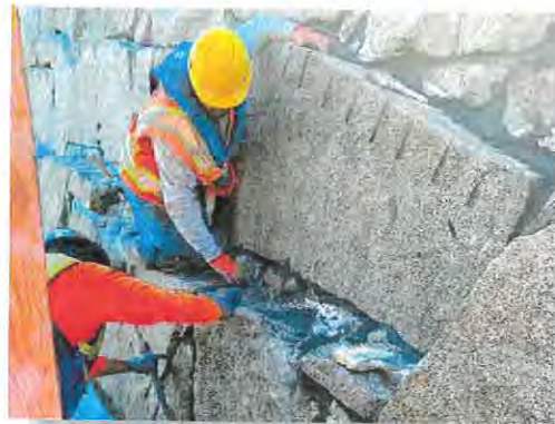
Grouting Stacked Rock – NCPA Union Dam
