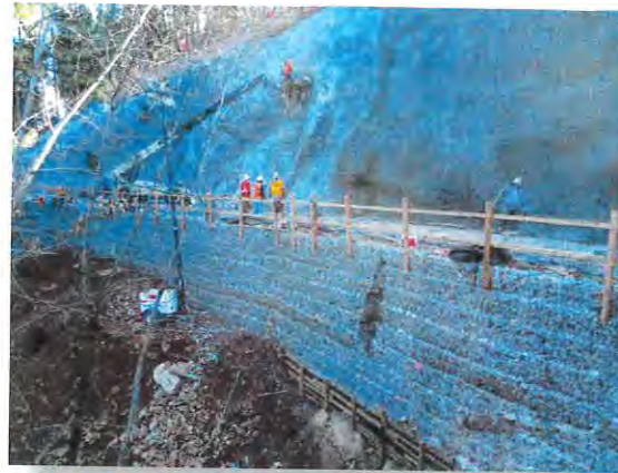
MSE Wall – Flume 51 Replacement
