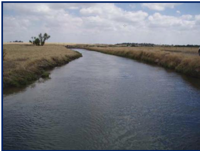
Figure 3-3. North Main Canal.
