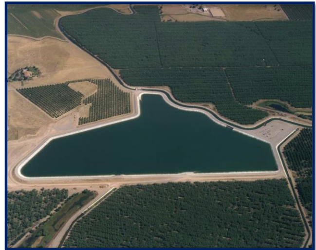
Figure 3-4. North Side Regulating Reservoir.
