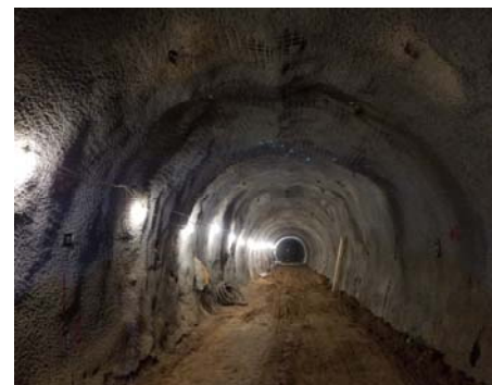
Inside of Tunnel
