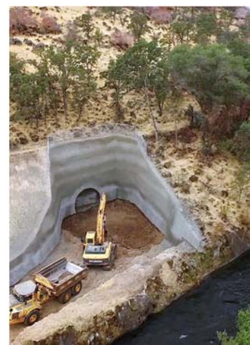
Upstream Portal of Tunnel
